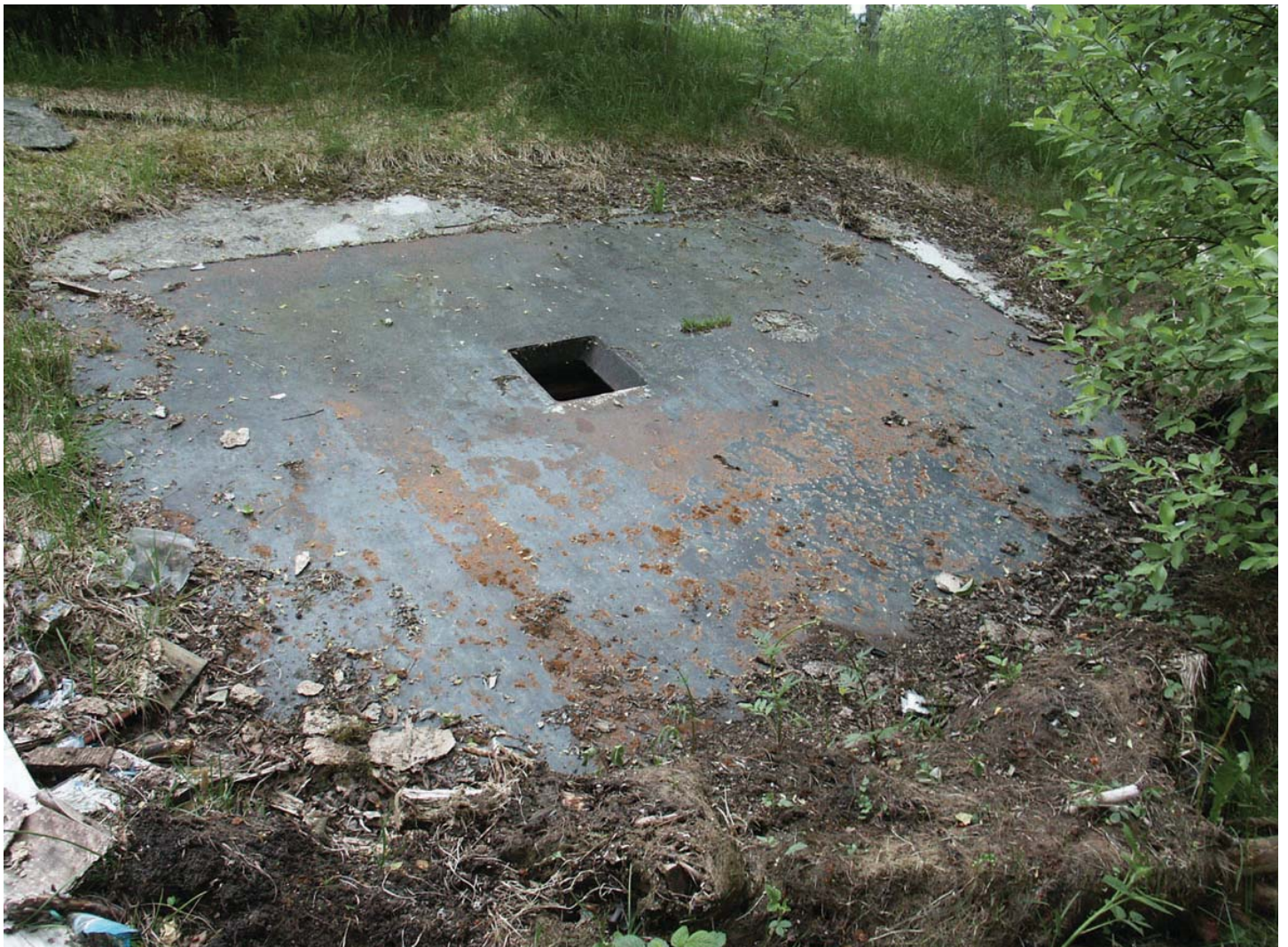
Steelplate 7P7 from outside
