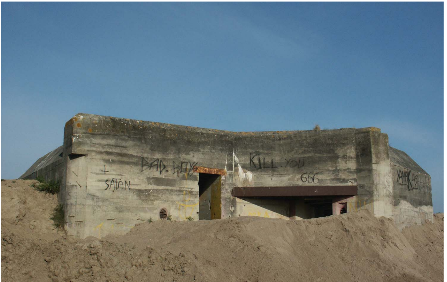
Entrance area of a R 143 in France - again different bunkertype with same task - artillery observation - here a steel-turret is used for observation, the entrance to the left lead to a Tobruk (MG-position)
