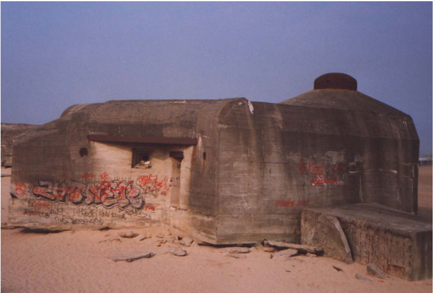
Entrance area of a R 120 in France - different bunkertype with same task - artillery observation - here a steel-turret is used for observation
