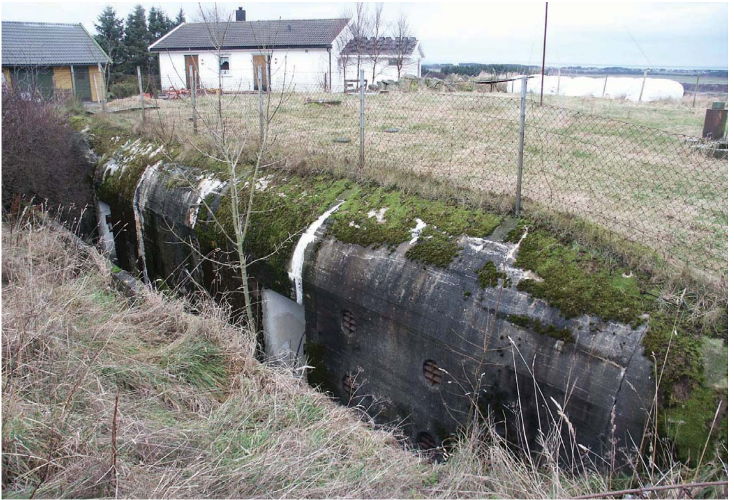
Lista Vestre Hauge: Entrance area of the Luftwaffe special-construction
