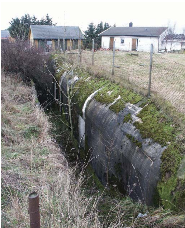
Lista Vestre Hauge: Entrance area of the Luftwaffe special-construction (different angle)
